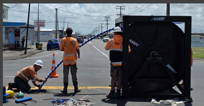
PULLING LINER INTO PLACE
